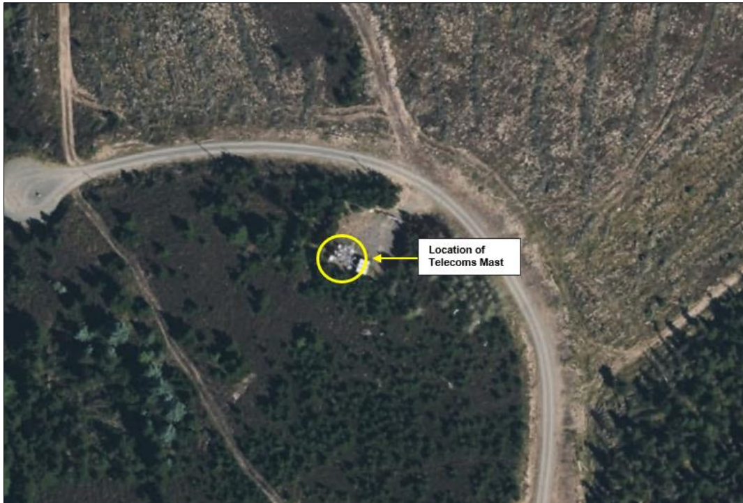
Figure 5. Telecoms Mast at VDF Ballydavid
