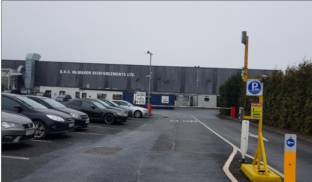
Figure 3. Telecoms Mast-site at B.R.C. McMahon Reinforcements
